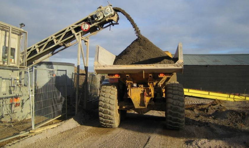
Placing of RCC in truck
