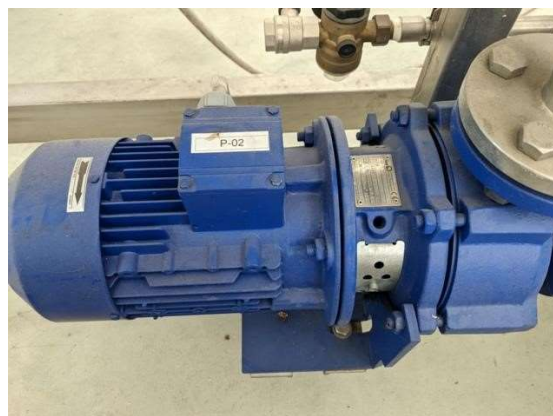
Figure 14 Centrifugal Pump
