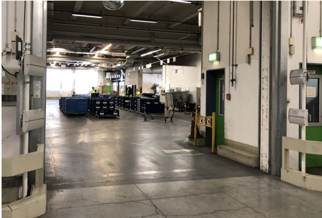
Figure 26 RFID gate installed according to guideline 2
