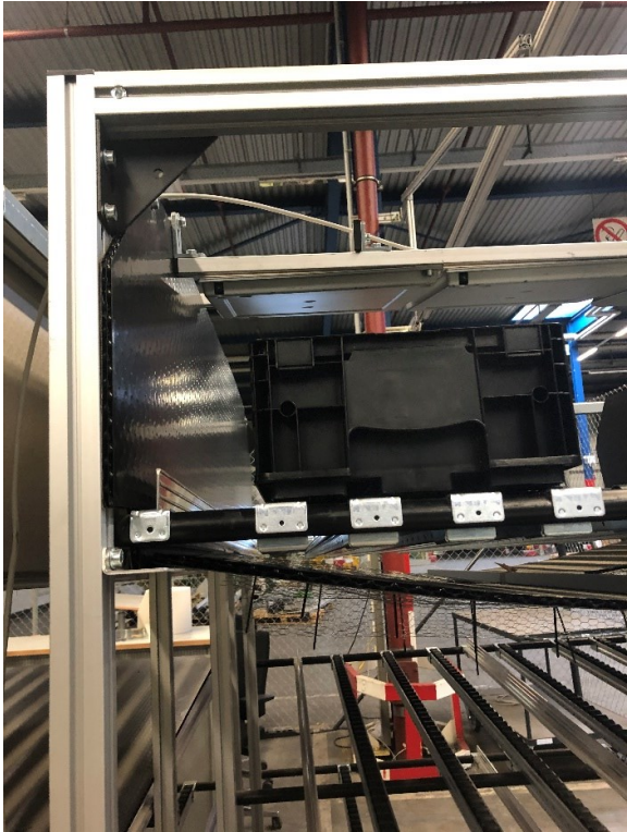
Figure 46 Setup of the RFID installation for the verification of the absorption test
