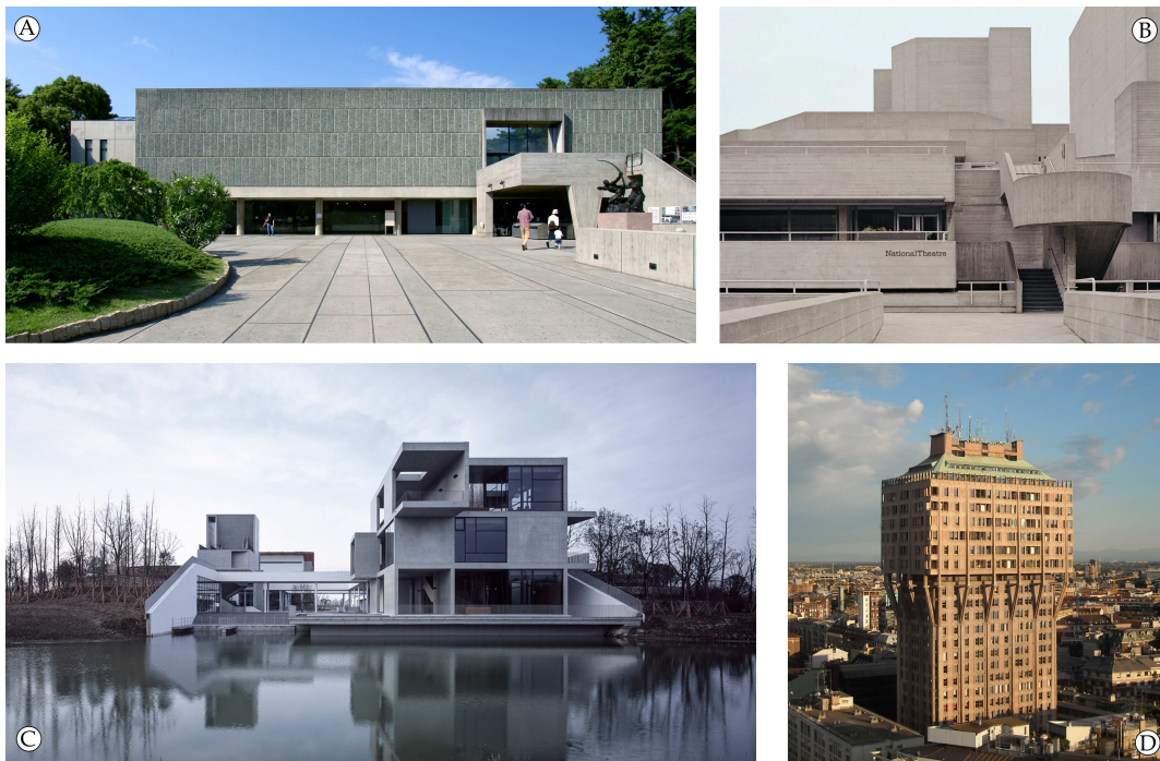
Figure 1.1: Usage of reinforced concrete in buildings. A) National Museum of Western Art by Le Corbusier, Tokyo, Japan; B) The Royal National Theatre by Denys Lasdun, London, United Kingdom; C) Suzhou Intangible Cultural Heritage Museum by Vector Architects, Suzhou, China; D) Torre Velasca by Studio BBPR, Milan, Italy.
