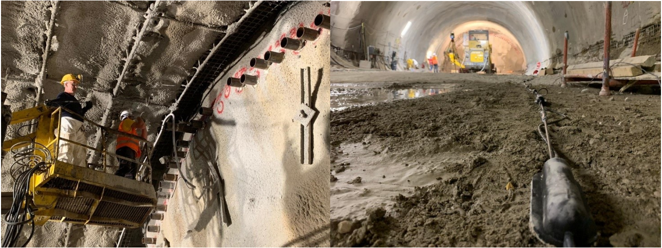
Figure 6.7 Left: Pre-Conv Array installation. Right: Pre-Conv Array preparation
