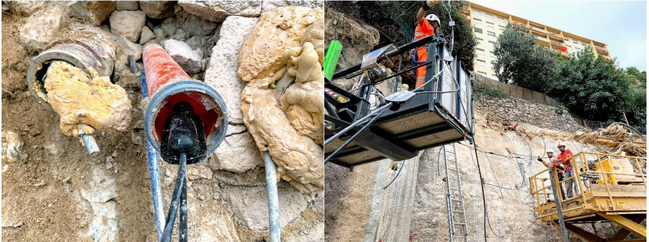
Figure 7.7 Pre-Conv Array installation procedure
