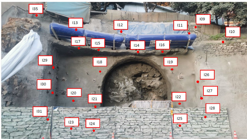
Figure 7.6 Geodetic survey on the tunnel entrance
