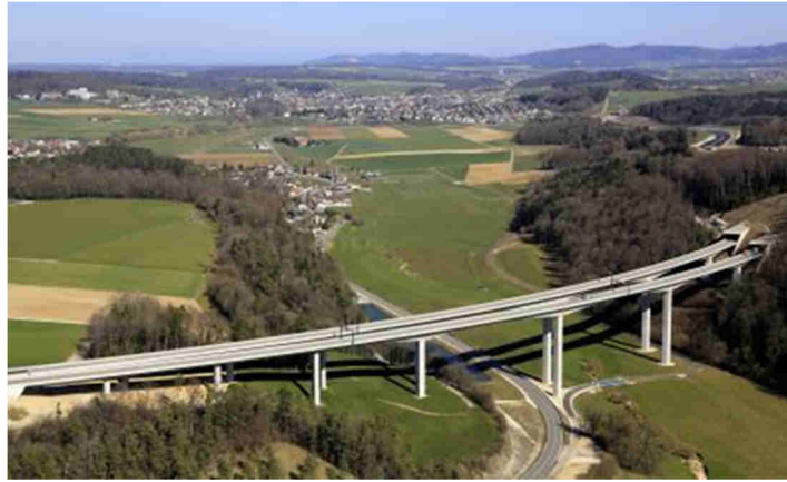
Figure 2.42: Longitudinal view of the bridge.
