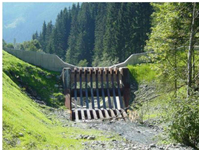
Figure 4.11: Slot grill barrier for dosing and filtering
