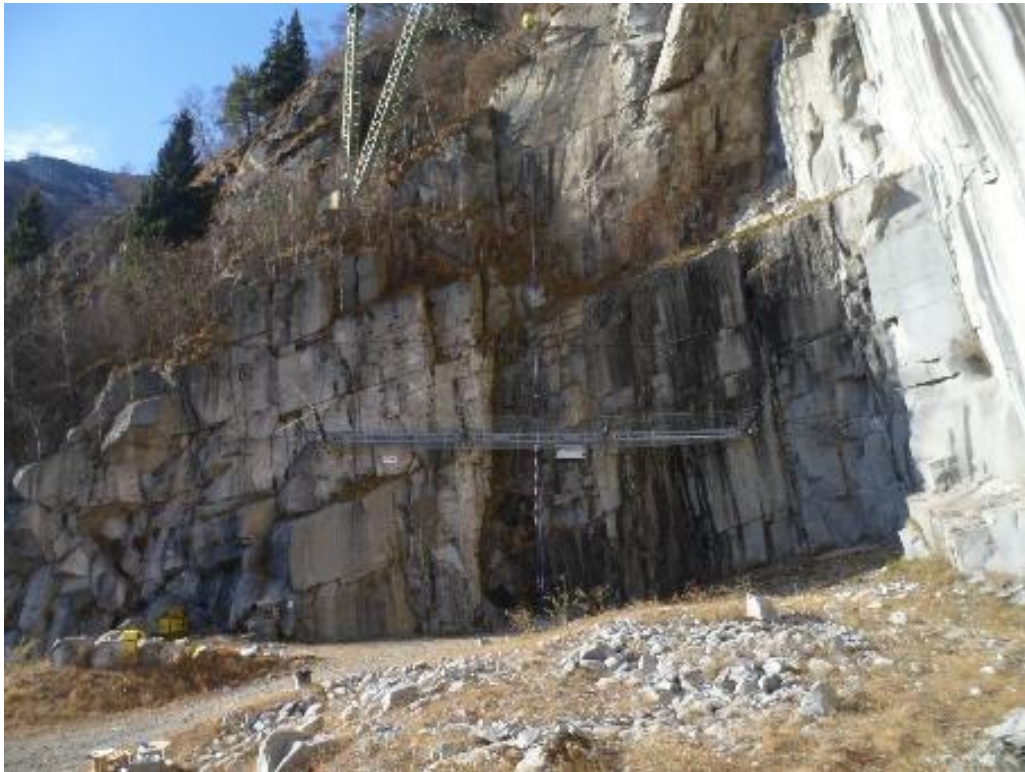
Figure 5.5: Installed kit on slope, overall view
