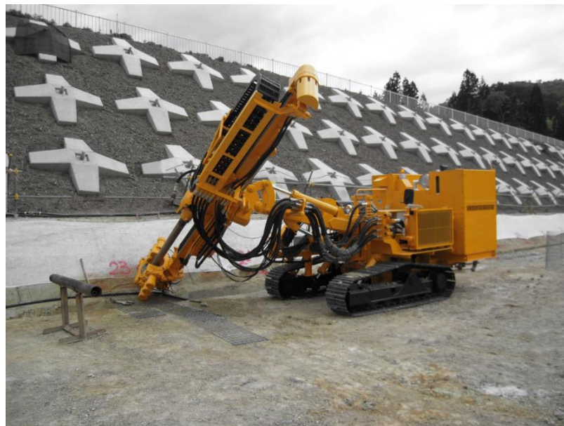
Figure 4.1: Slope stabilization anchor work for landslide prevention
