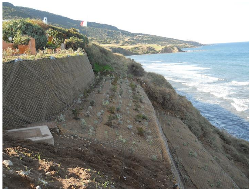
Figure 4.8: Consolidation intervention made by mono-anchorage umbrella structures combined with soil bioengineering
