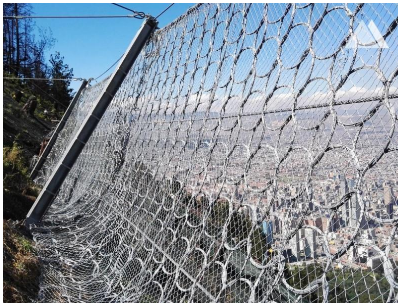
Figure 4.41: Combination of wire ring mesh panel and secondary net
