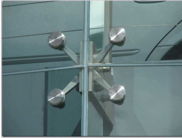
Figure 6.4: Detail of the supporting points.
