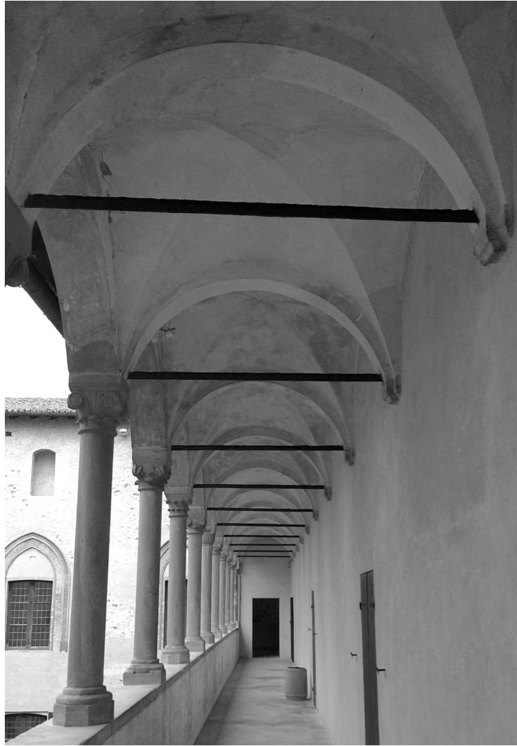
Figure I.1. Tie-rods in the Castle of Torrechiara in Langhirano, Parma, Italy.
