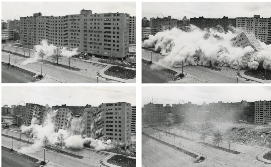
Figura 29 - Pruitt-Igoe, Saint Louis, US, (Fonte: U.S. Department of Housing and Urban Development, The second, widely televised demolition of a Pruitt-Igoe building that followed the March 16 demolition, immagini non coperte da Copyright riportate su Wikipedia )
