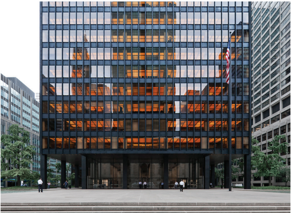
Figure 3.4. Seagram Building, New York, 1954-58. Architect: Ludwig Mies van der Rohe.
