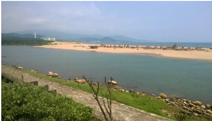
Figure 1.1 - In the upper left corner it is possible to notice the Lungmen power plant in northern Taiwan (credits: Stocchi).
