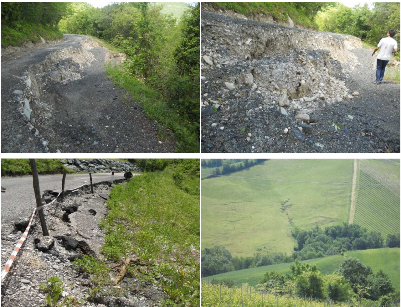
Figure 4.6 Photographs of some landslides surveyed in Calestano.
