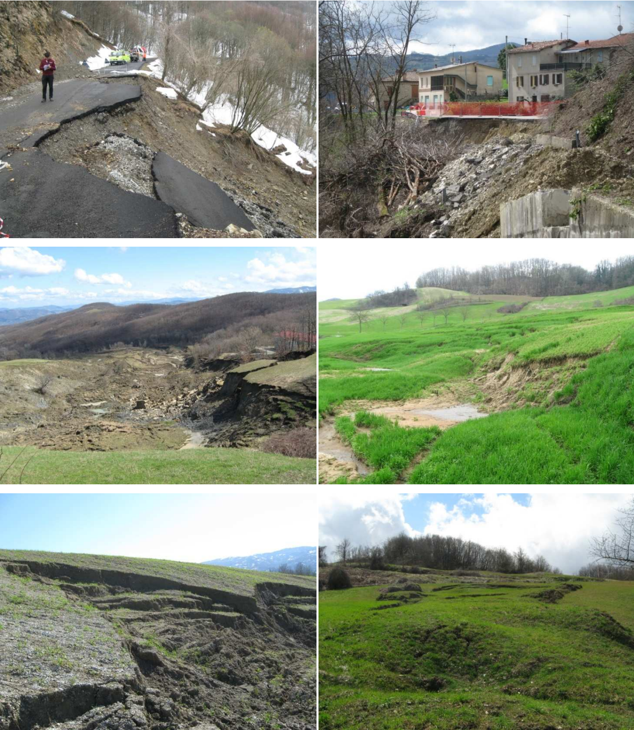
Figure 4.11 Photographs of some landslides surveyed in Tizzano Val Parma.
