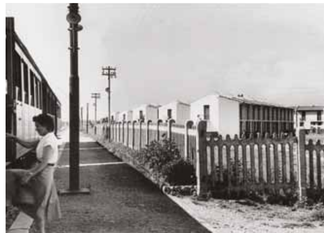
The alienation of the Italian Modern city. Frame from the movie La notte , Michelangelo Antonioni director, 1961 and Ina-casa Residential district Cesate (Milan) by architects BBPR, Franco Albini, Ignazio Gardella, and others, 1950-1954.
